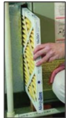
Figure 11: Remove all air filters
