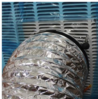
Figure 18: Flex Duct connected to the Flange.
